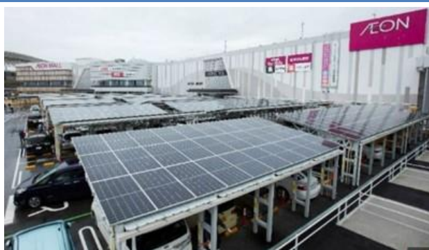
Figure 22: Progressively installing more solar PV panels across AEON malls
